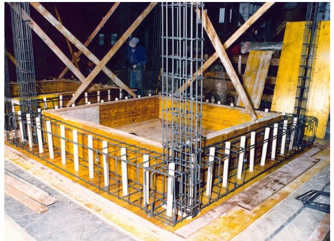
Fig. 4. Detail of the reinforcement.
